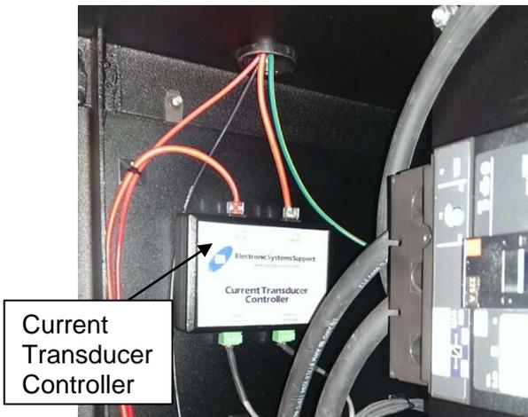
**5.2.6.** Connect the 7ft. red RS-485 cable to the RS-485 connector on the Current Transducer Controller labeled "RS-485 OUT". Feed this cable through the bushing located on top of the battery cabinet and connect it to a RS-485 connector on the Ambient Temperature Probe labeled "RS-485 IN".
